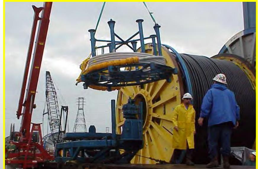
King used Standard baskets and was transported without permit making this an ideal method for up to 6 flying leads
